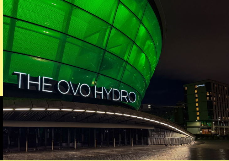
Right: The Ovo Hydro Arena in Glasgow, Scotland. Below: The basalt lava facade of Mumok museum Vienna, Austria.
